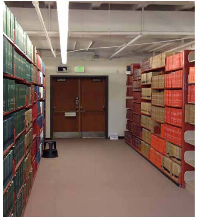
Existing Separation at Klamath Hall Basement from Library under Cascade Hall. An alarmed exit door connects to an enclosed stair that leads to ground level.
